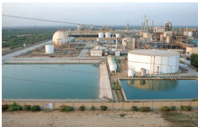
Evaporation Pond at Plant Site
