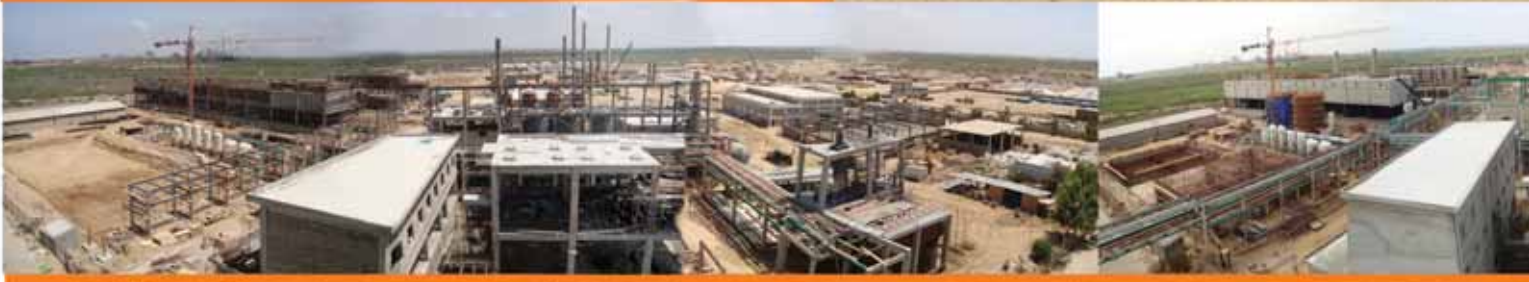
EPCL Project during different phases of construction
