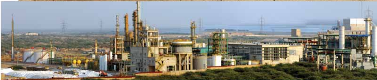
EPCL site on completion of Project
